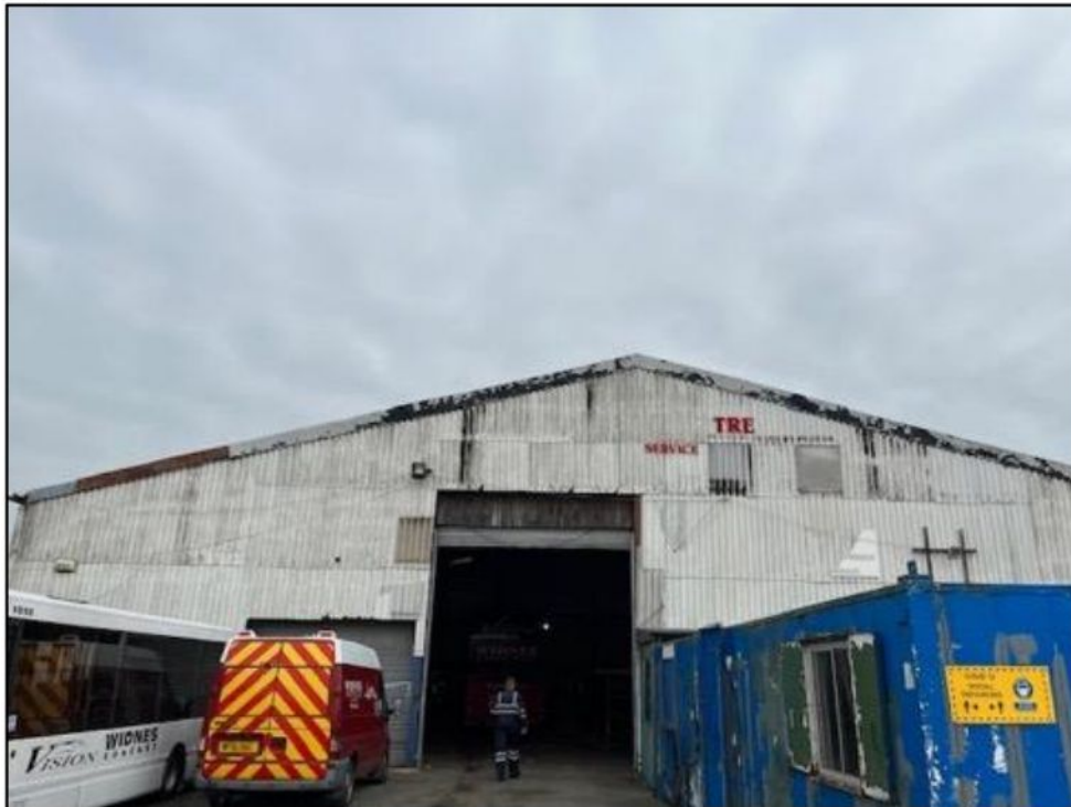
Photograph 1: A front view of the large corrugated storage/workshop building.
