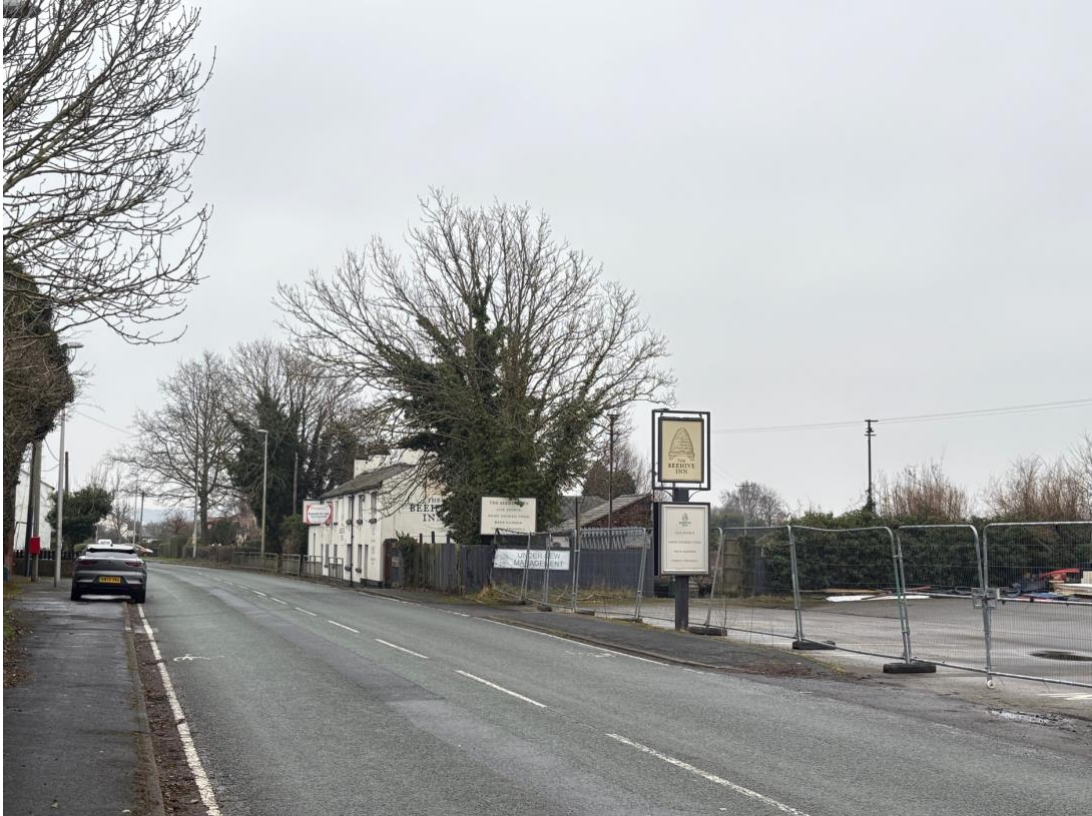
Figure 10- Beehive and car park from the west
